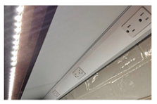
Under Cabinet Lighting & Plug Mold
