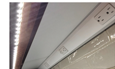
Under Cabinet Lighting & Plug Mold
